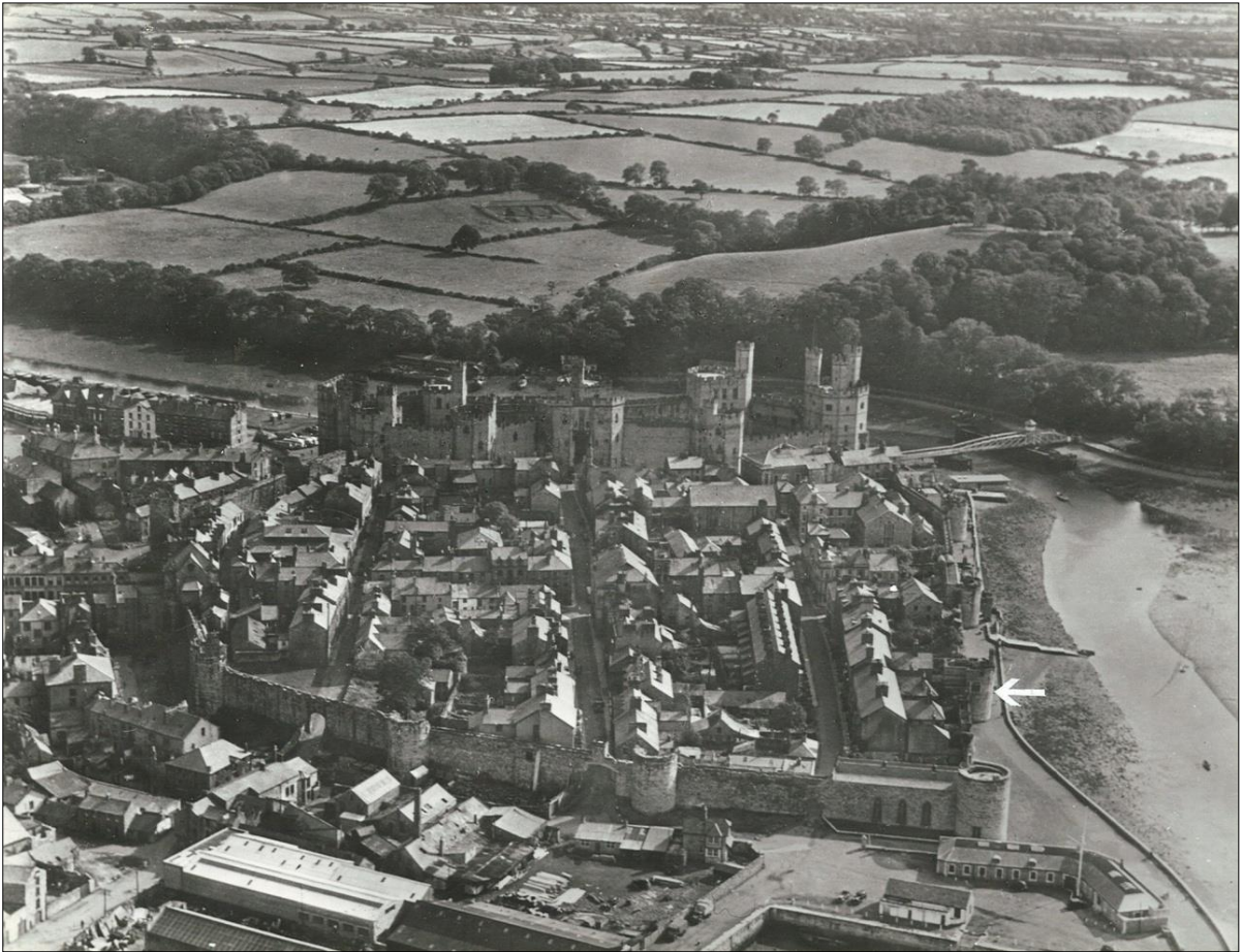
An aerial view of Caernarfon Castle and Town Walls Showing the Position of the Bath Tower – Aerofilms Ltd (c. 1960s)
