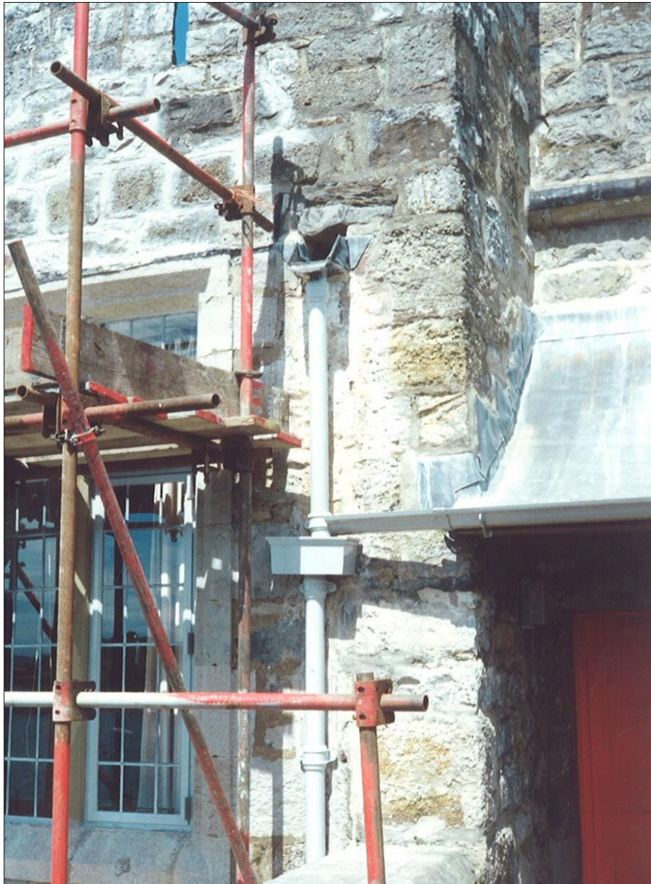
Restoration Work to the Masonry of the Bath Tower (c. 1983)
