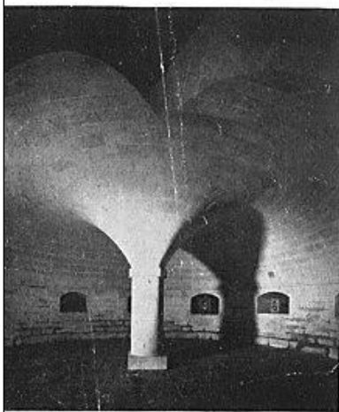
8.—THE MAUSOLEUM UNDER THE CHAPEL
