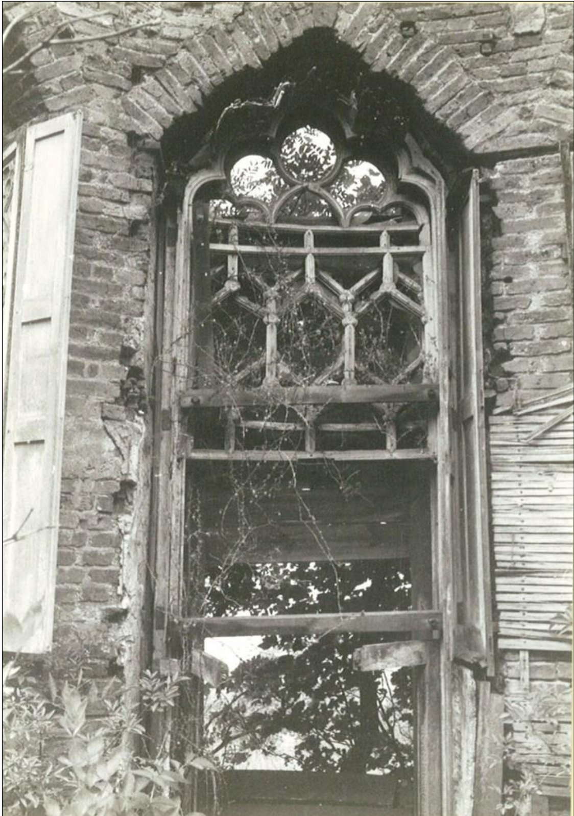
Very little of the old window frames or sashes could be reused but the new ones are exact copies.
