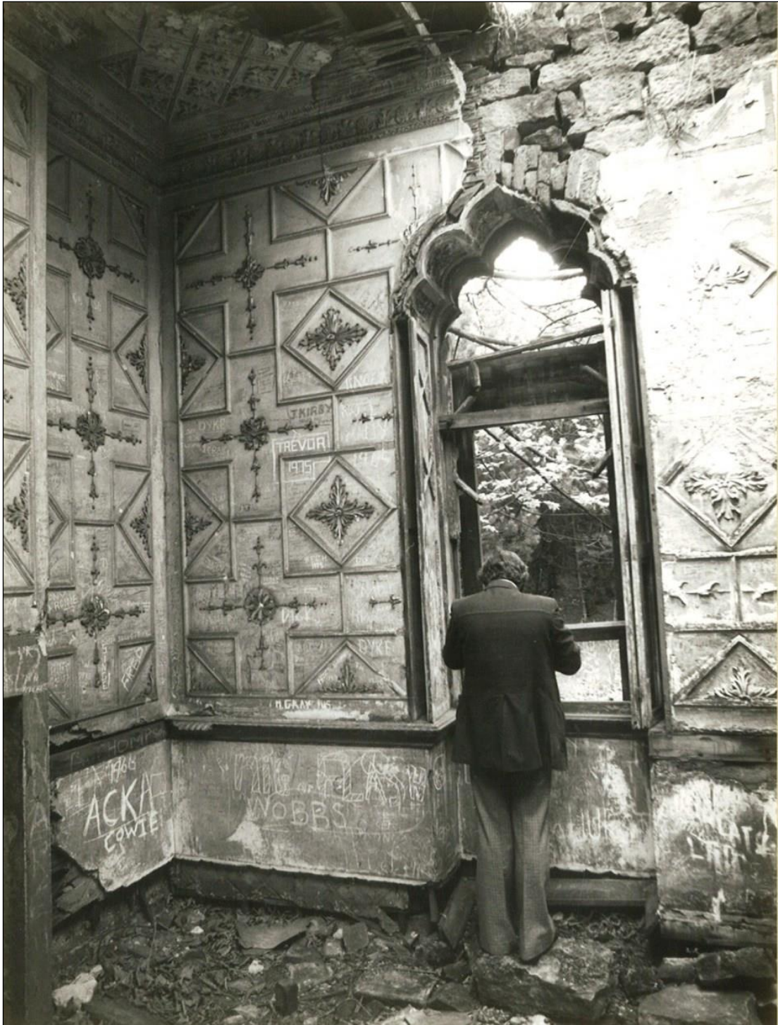
The carved timber dado rail in the bedroom can be seen on the left. It was copied for the Banqueting Room, but left plain in the bedroom.
