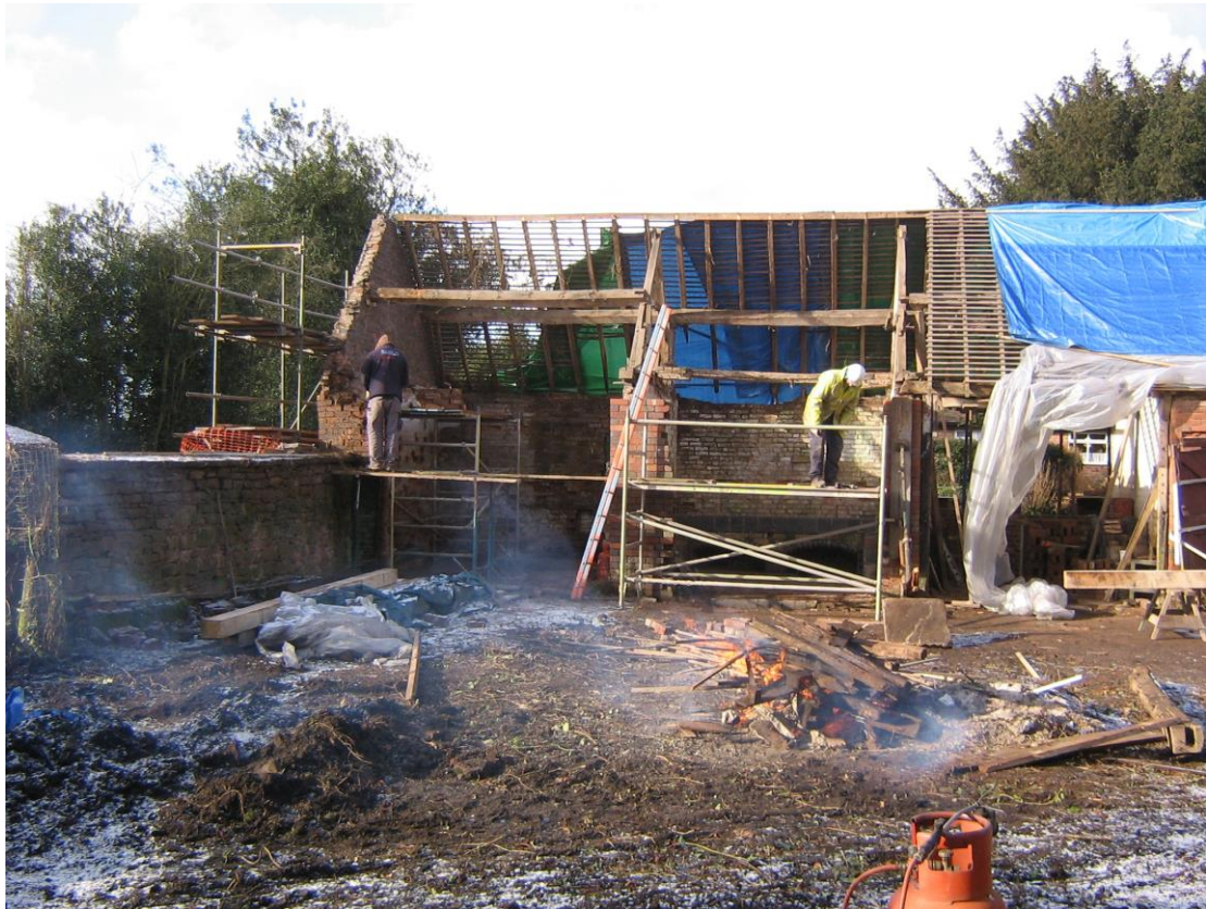
The sheds being re-roofed and the end gable rebuilt.
