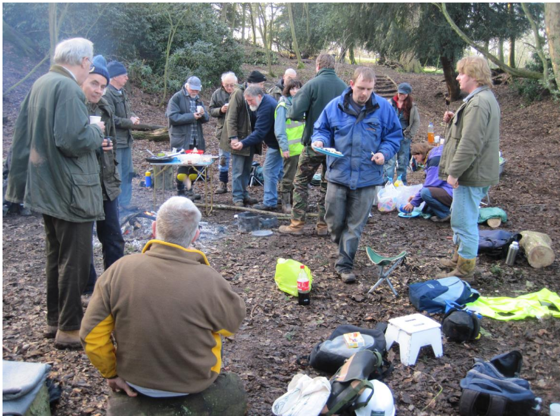
Volunteers clear the holloway, Dark Lane (above) and take a well earned break (below).
