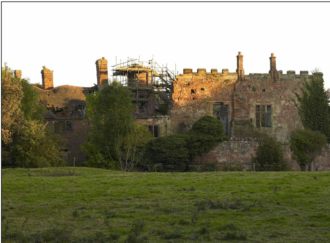
East (top) and west elevations of Astley Castle in September 2007. Note the brick skin of the vice tower still partially standing in the centre below, and the northern portions of the castle that could not be saved and had to be taken down.
