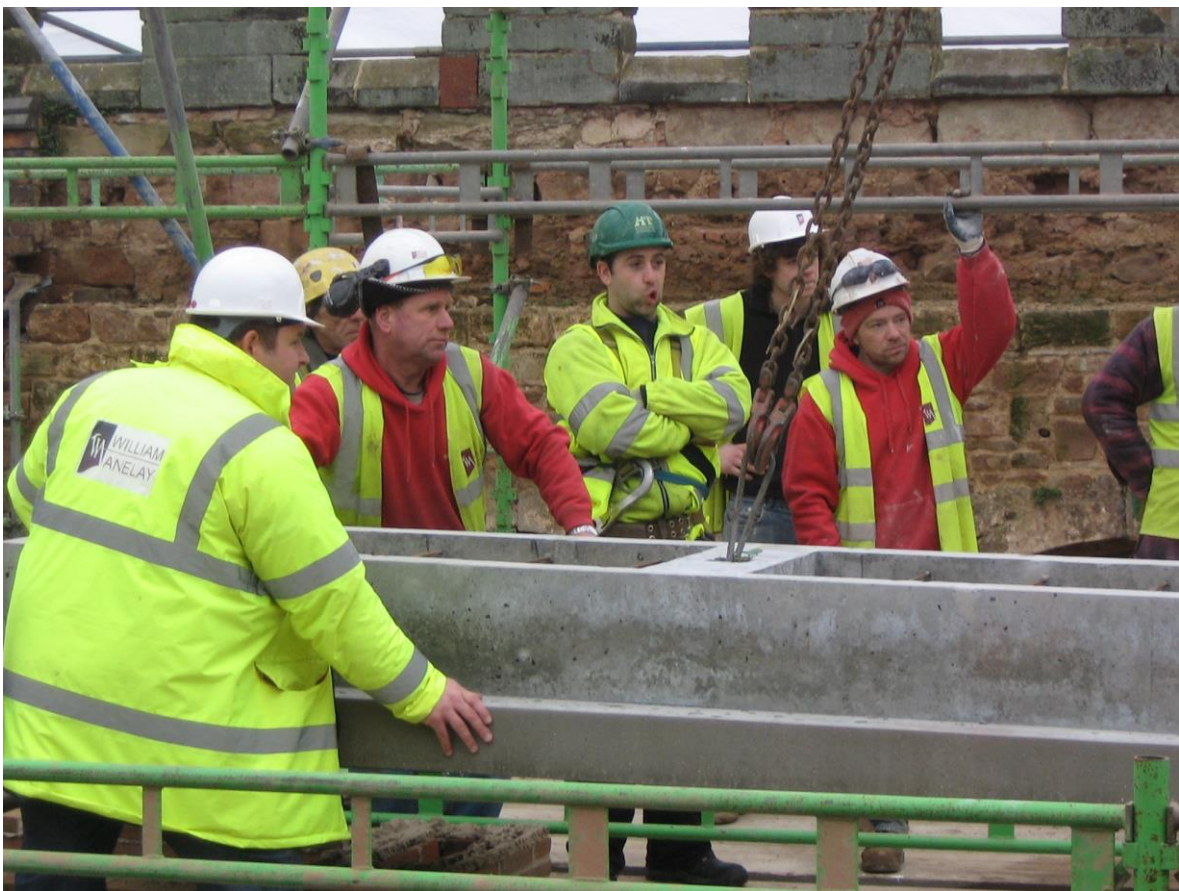
The lintel was lowered into position with millimetre precision
