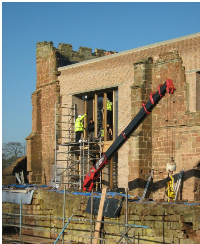
Fitting the double-glazed units using a crane with suckers
