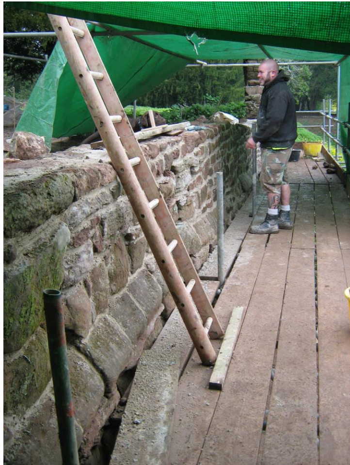
The rebuilt curtain wall close to its finished height
