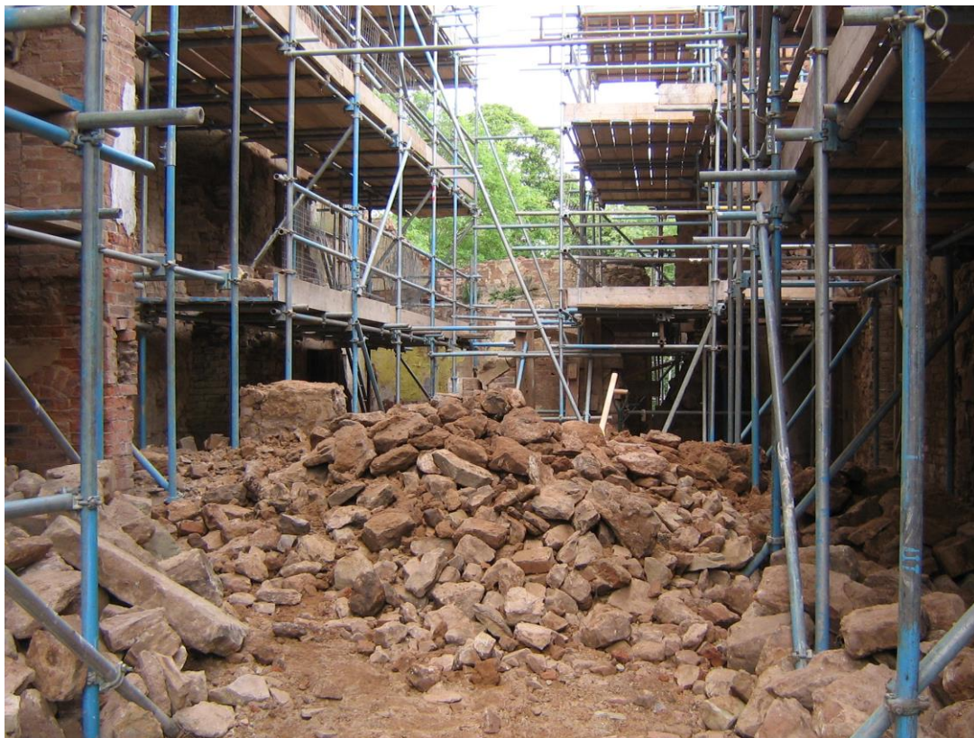
The cross wall on the ground floor being demolished
