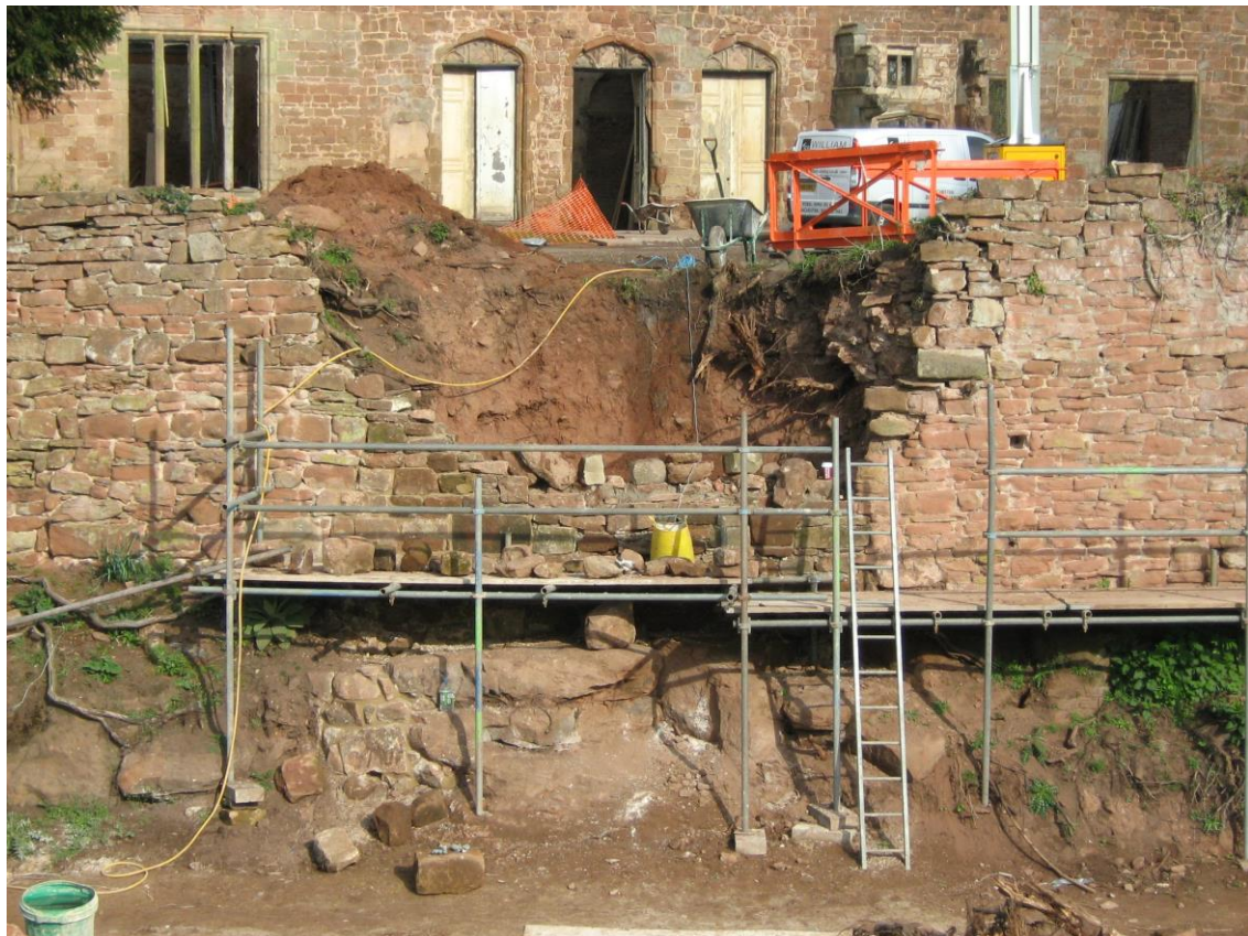
Two areas of the curtain wall on the east side had completely collapsed
