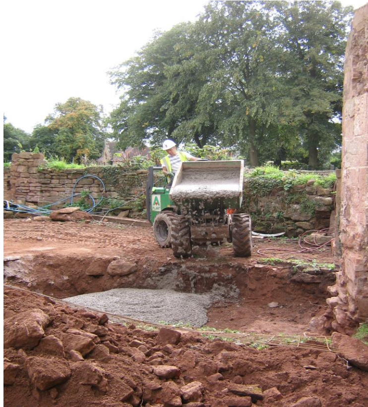
Concrete footings going in for the new diaphragm walls
