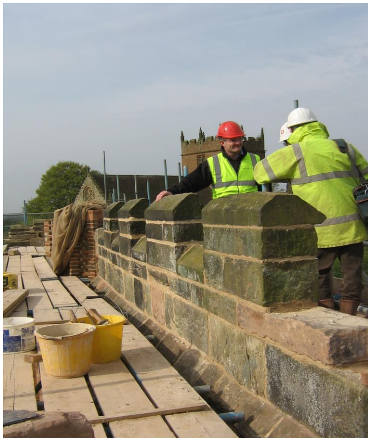
A significant area of the west wall had to be taken down and rebuilt
