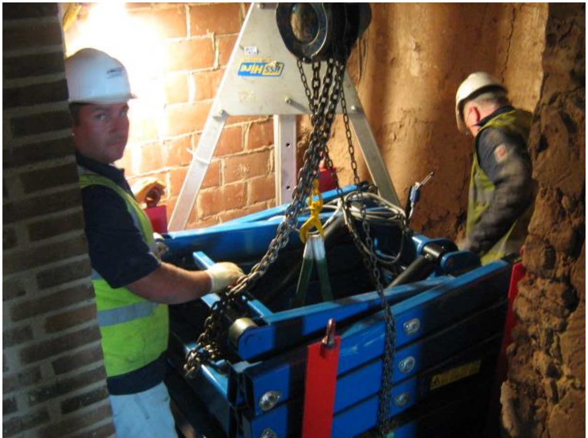
The scissor mechanism for the lift being lowered into its pit
