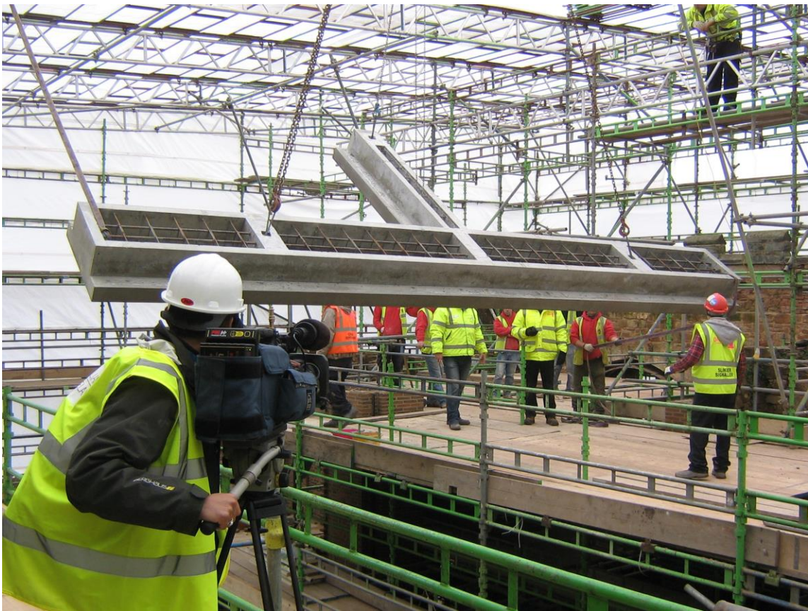
The heaviest T-shaped lintel being lowered through the roof
