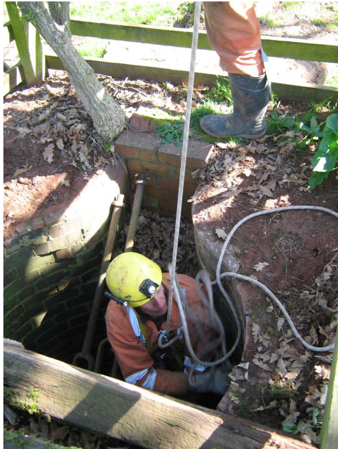
Mark Noble of Geotechnical prepares to go down the well 15 metres down there was a blockage but water was discovered below this. The old pump mechanism is visible
