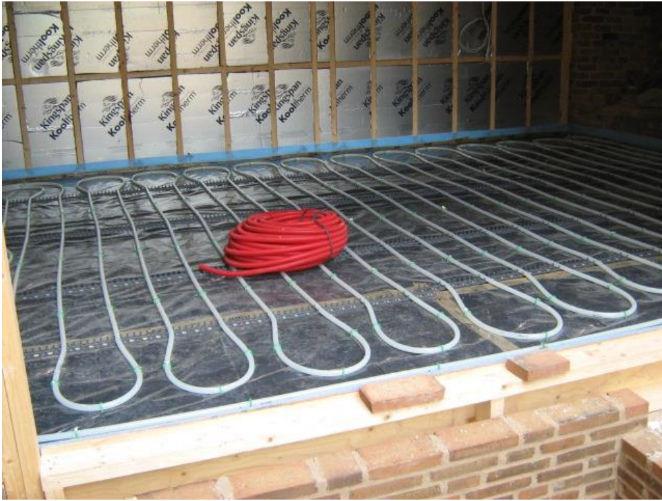
Underfloor heating pipes going in
