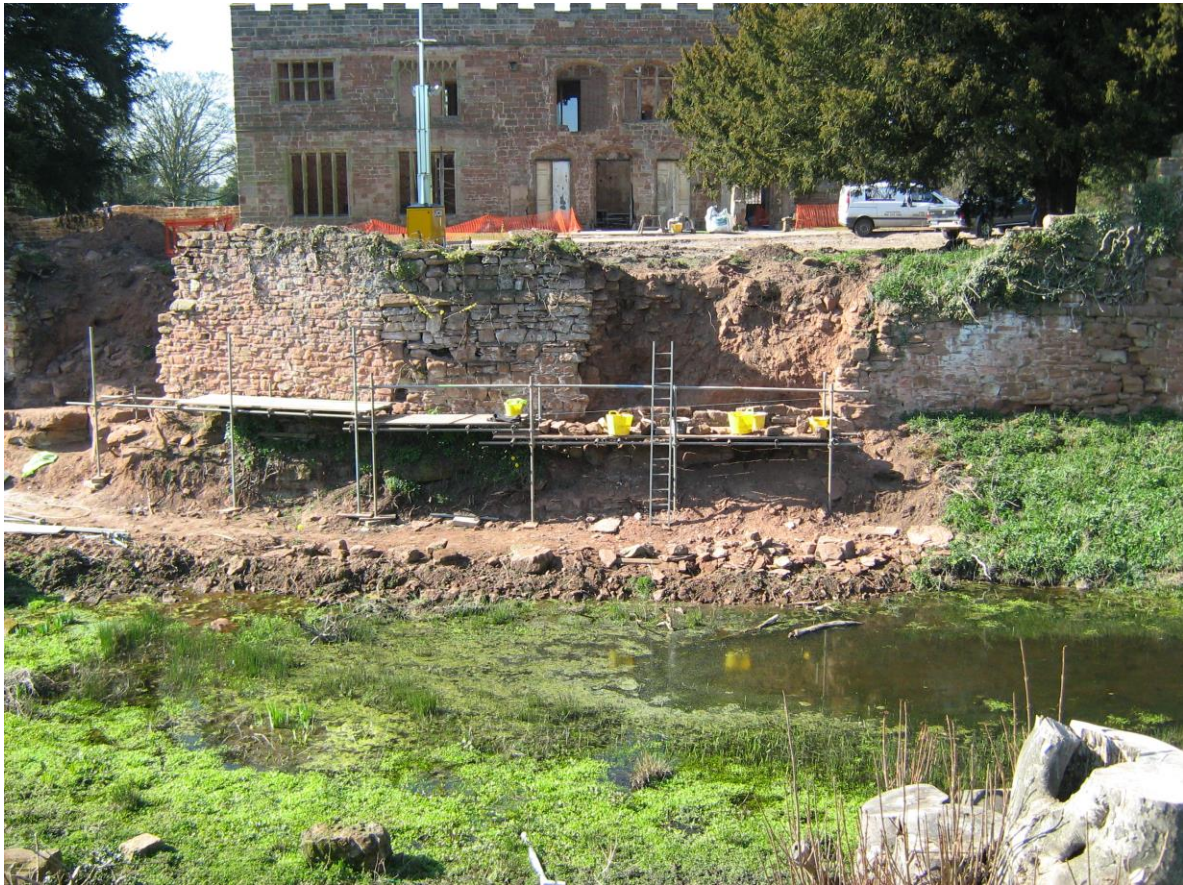
Two areas of the curtain wall on the east side had completely collapsed
