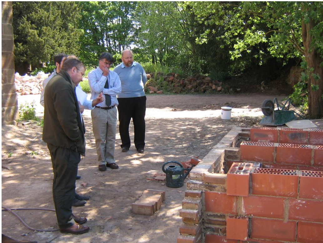
A sample section of the proposed diaphragm wall showing the use of clay blocks
