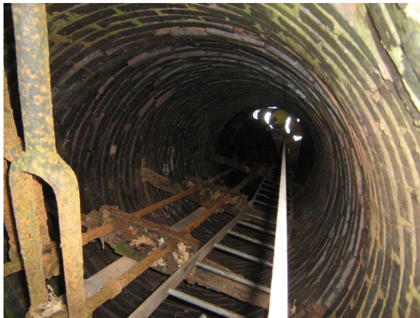
Mark Noble of Geotechnical prepares to go down the well 15 metres down there was a blockage but water was discovered below this. The old pump mechanism is visible
