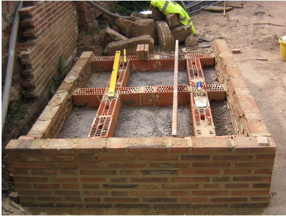
A sample section of the proposed diaphragm wall showing the use of clay blocks
