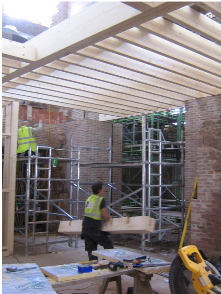
The ground floor ceiling going up
