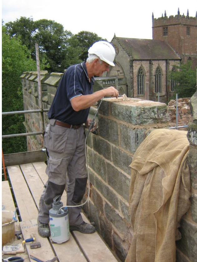
Len Hardy rebuilding the merlons on the east elevation
