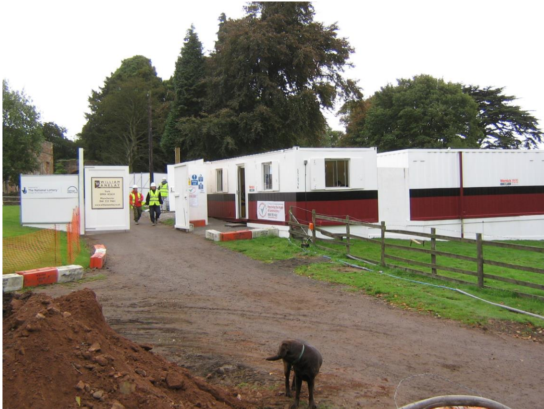
Anelays' site compound on the way up to the moated site
