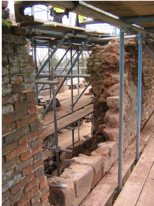
A significant area of the west wall had to be taken down and rebuilt
