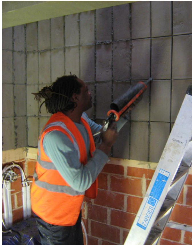
Grouting up the tiles to the kitchen niche
