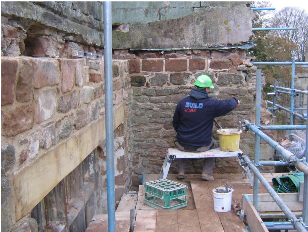
Ian McGregor of Buildright repointing the garden court walls
