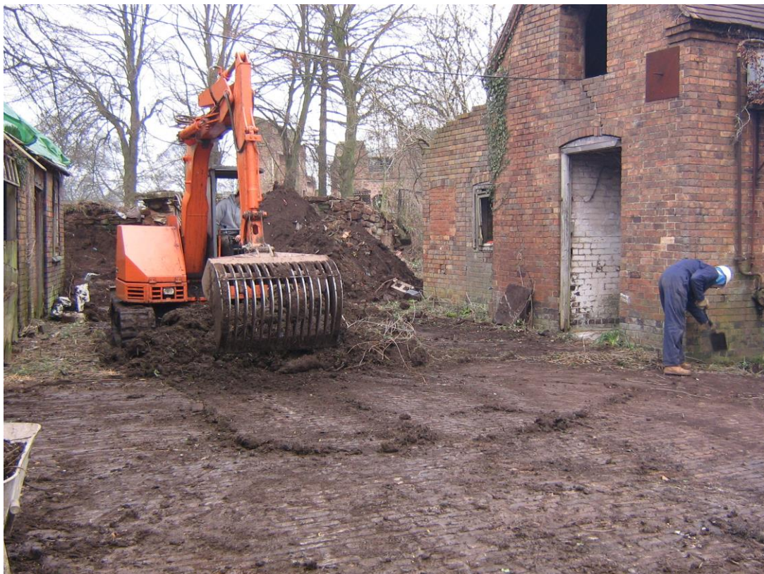
Clearing the Coach House yard and finding the brick paving
