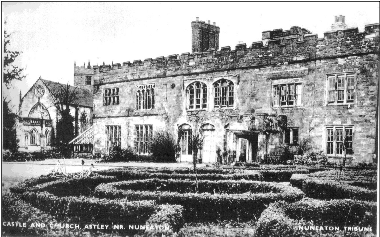
Astley Castle before the War. Note too the castellated vice tower showing above the crenellated parapet.
