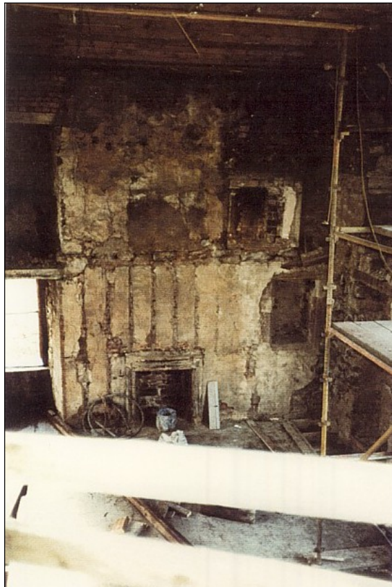
Stripping out Victorian partitions as work began.
