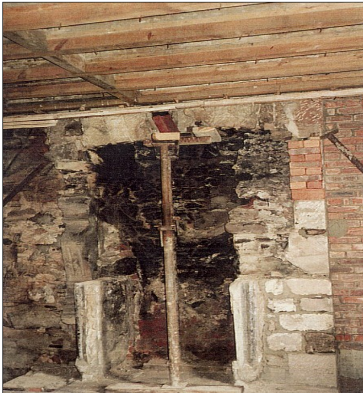
The great hall fireplace, with a later one below it, showing that the floor level was lowered, probably in the later 17 th century.
