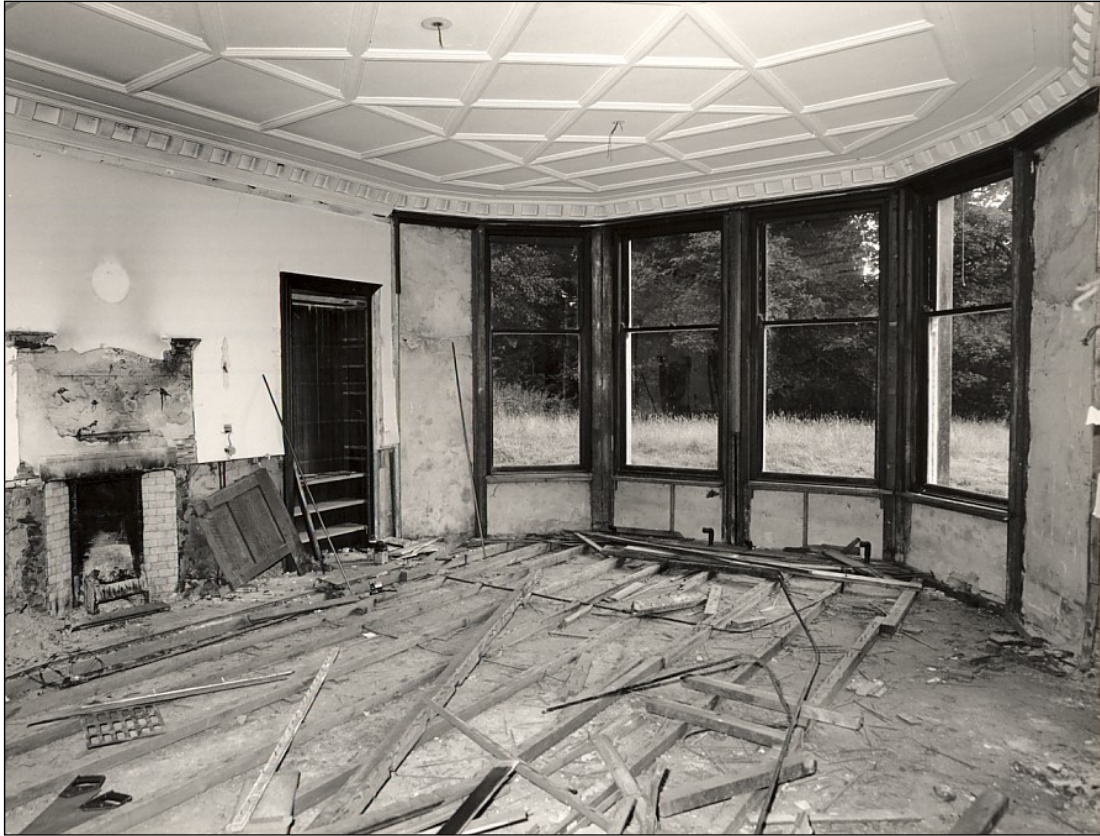
The late Victorian drawing room in 1989 (now demolished).
