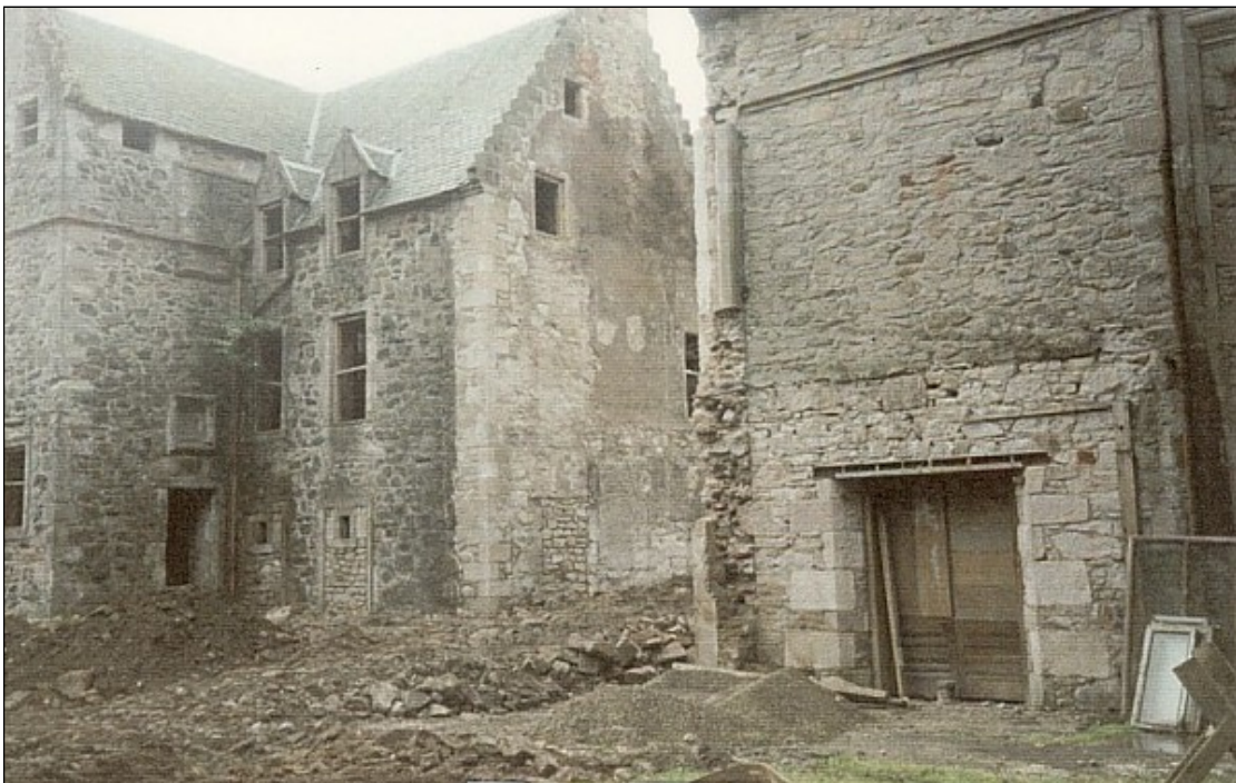
Demolitions complete. The ground is being restored to its old level.
