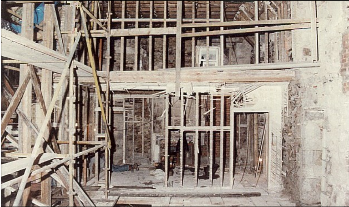
Stripping out Victorian partitions as work began.
