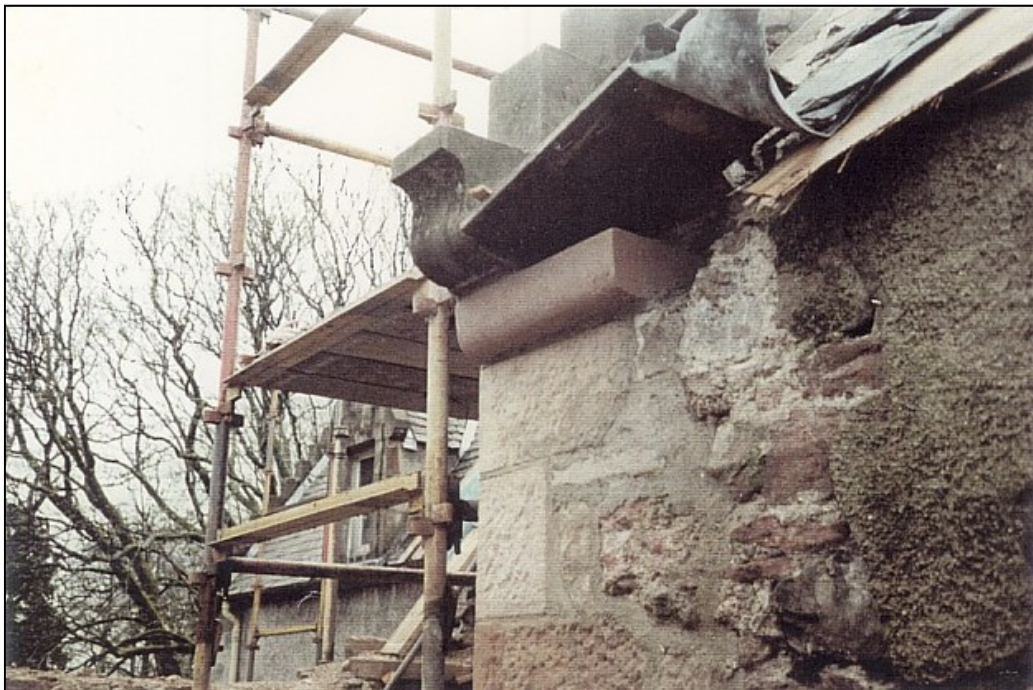
Crowsteps being put back on the North gable.
