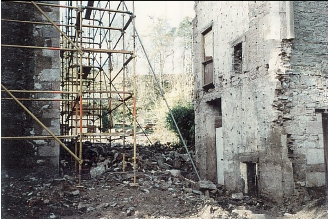
The stair tower separated, but with its south wall unfinished.
