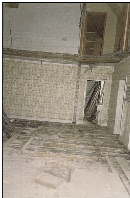
The main floor, looking north.
