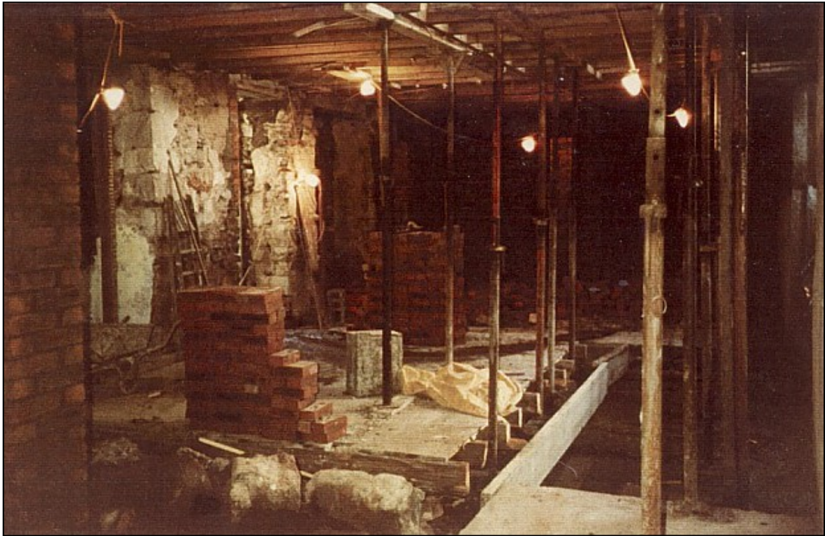
Holding the building up while work starts.
