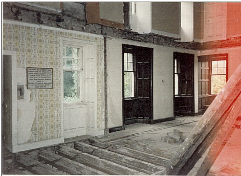
Inside the house in 1986 before restoration – the main floor looking east.
