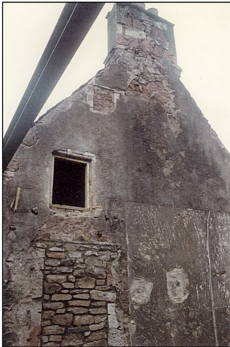
North gable without its crowsteps. They had been removed when that side was extended.
