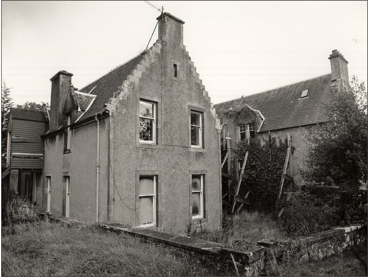
The 19 th century west wing, now demolished, with the old house beyond it, its west well shored up. Photograph taken in 1989.
