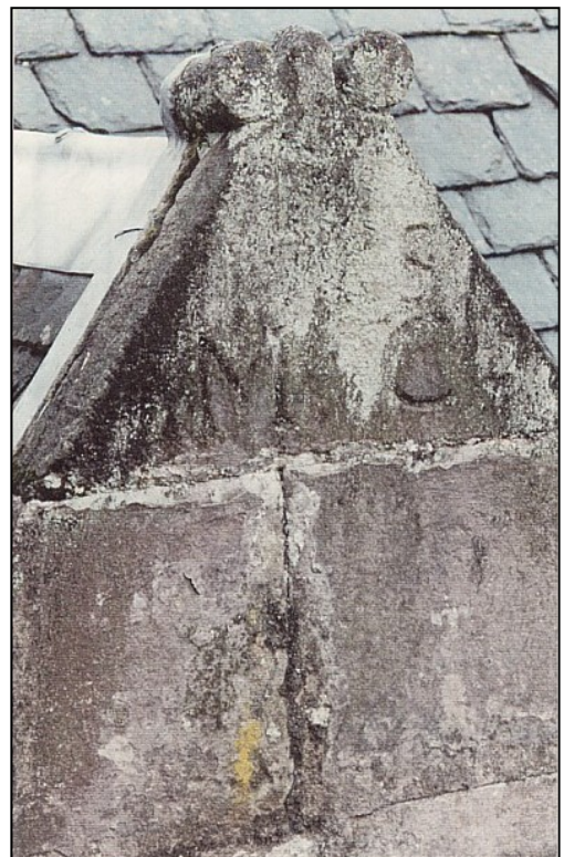
The dormer with the carved initial before clean up.
