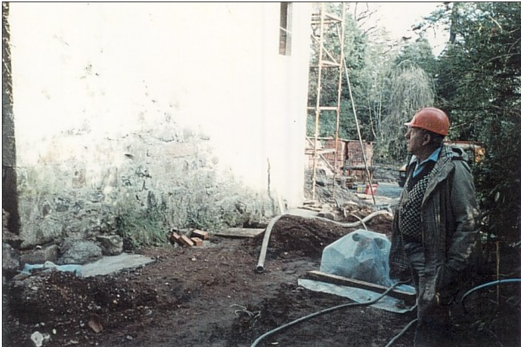
The south wall, where the foundation stones were showing.
