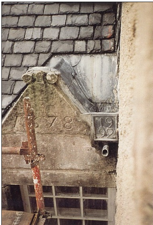
New rainwater spout – the old drainpipes have gone.
