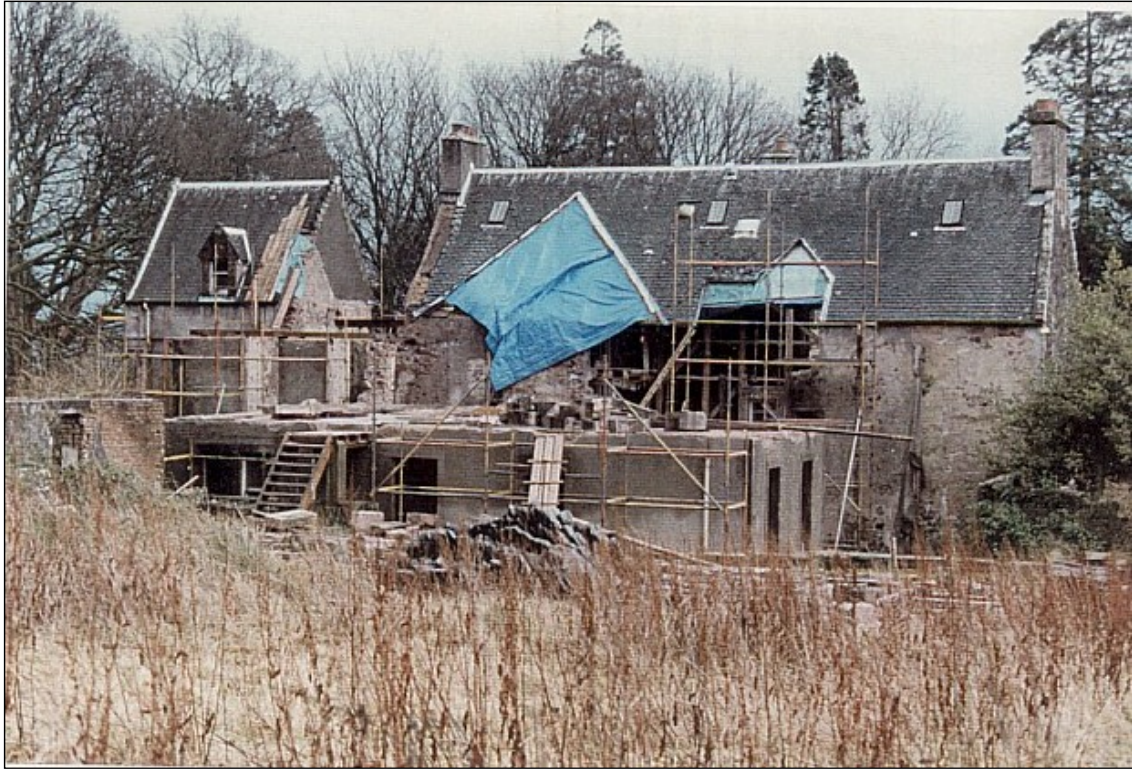
The west side during demolition.
