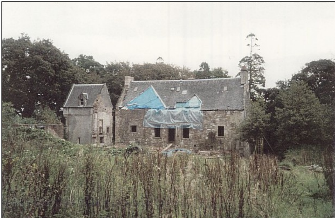
The west side remodelled, with the "discovered" windows at each end.
