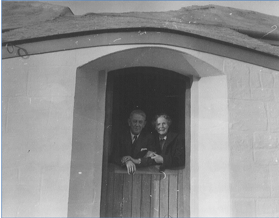
Donald and Viva Thomas, leaning on the new door of their cottage on completion of the conversion in 1957.
