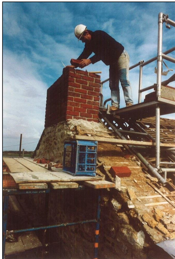
Rebuilding the chimney of the new cottage.
