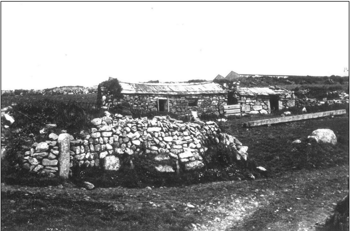
Early house and shippon (cattle shed) at the top of Lower Porthmeor, known as Grace's House. The enclosure in the foreground was a garden.
