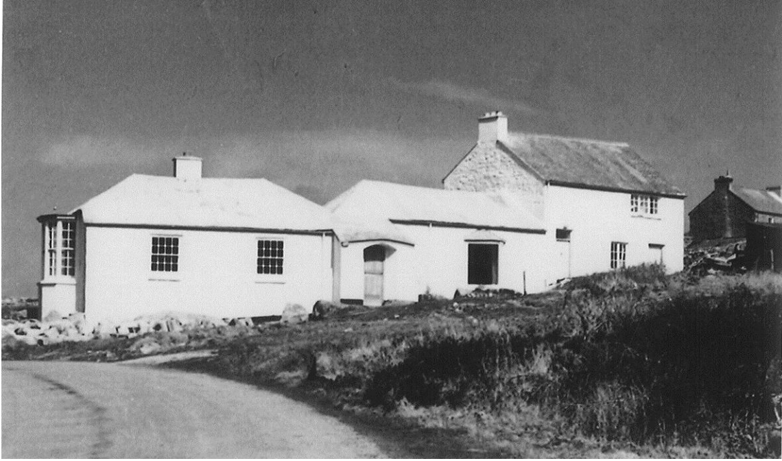
Arra Venton in 1957 after D.W. Thomas's remodelling.
