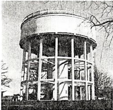
13. Larger tank — structure gets out of hand.
