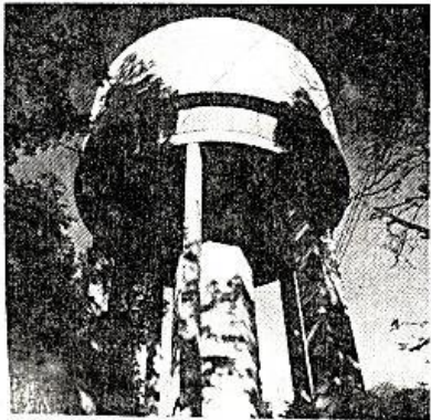
14. Structure simplified into highly stressed fins.
