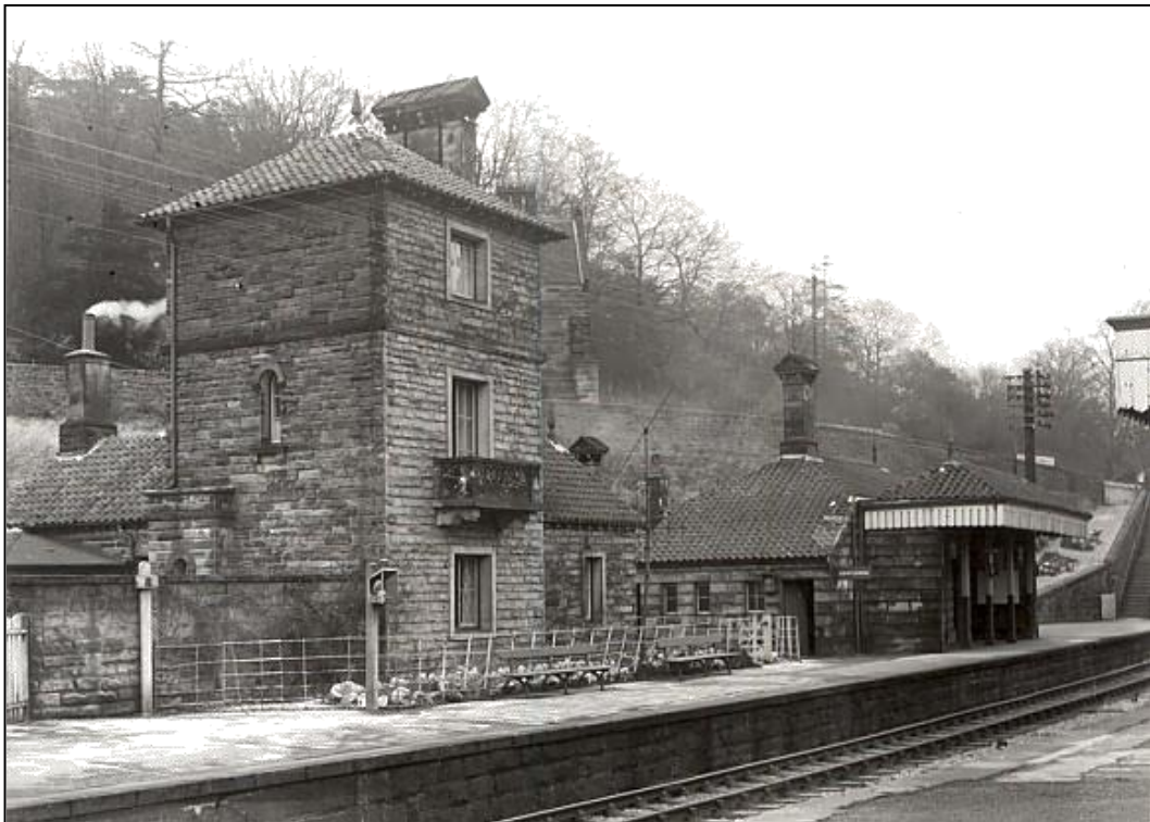
The last Station Master continued to live in the house after the station had been sold by British Rail.
