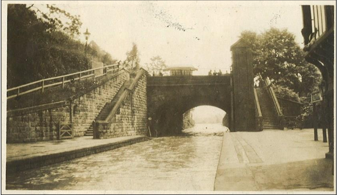
Alton Station railway track flooded in 1927 (photos from Graham Eyre).
