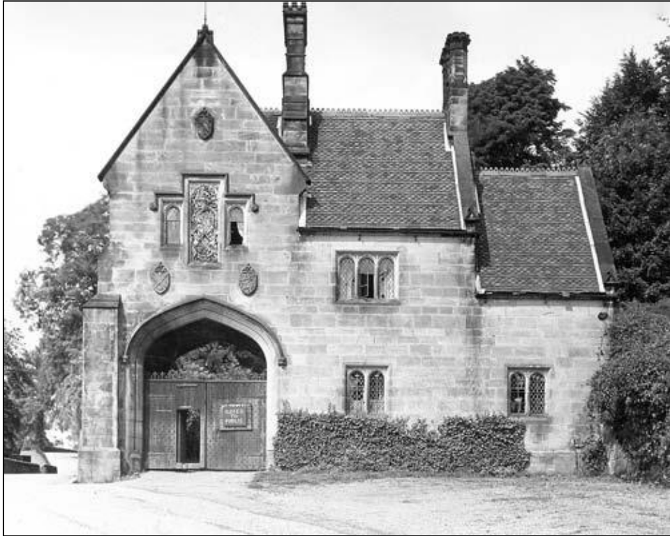
Station Lodge, designed by Pugin about 1849
