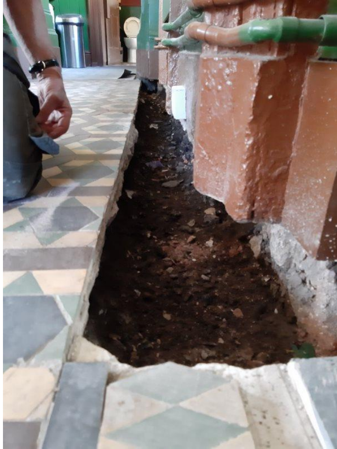
Burying unsightly pipework in the Waiting Room.
