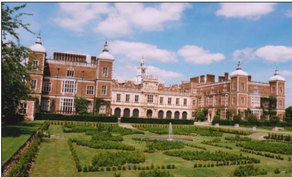
The south elevation of Hatfield House showing the open loggia, portico (with an attempt at Classical orders), Flemish gables and lantern, all of which may have been references for Campden House.
