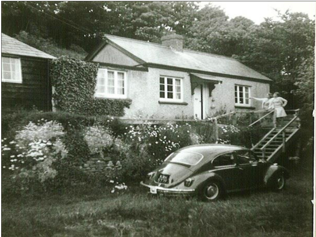
Chapel Cottage before restoration
