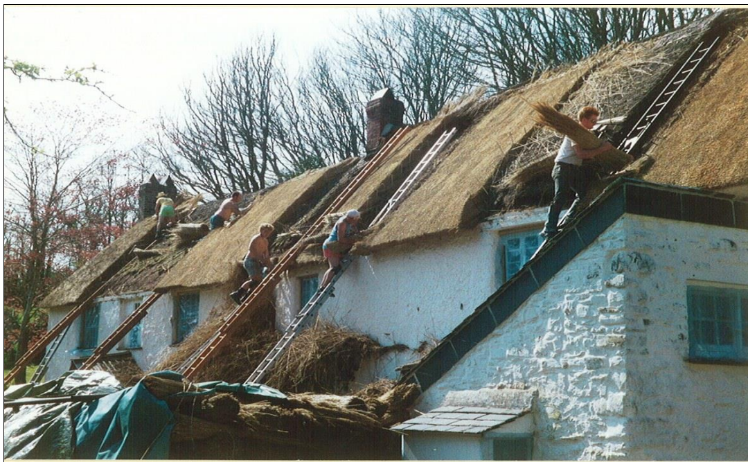
Re-thatching at Hawker's cottage
