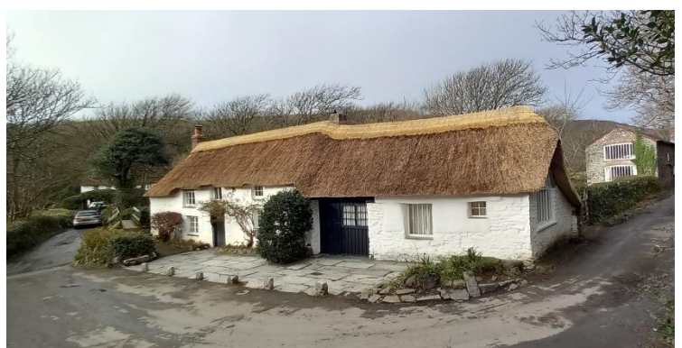
The thatch before (top) and after repair. As the front slope was in still good repair there was no need to renew it, apart from the protective ridge.
