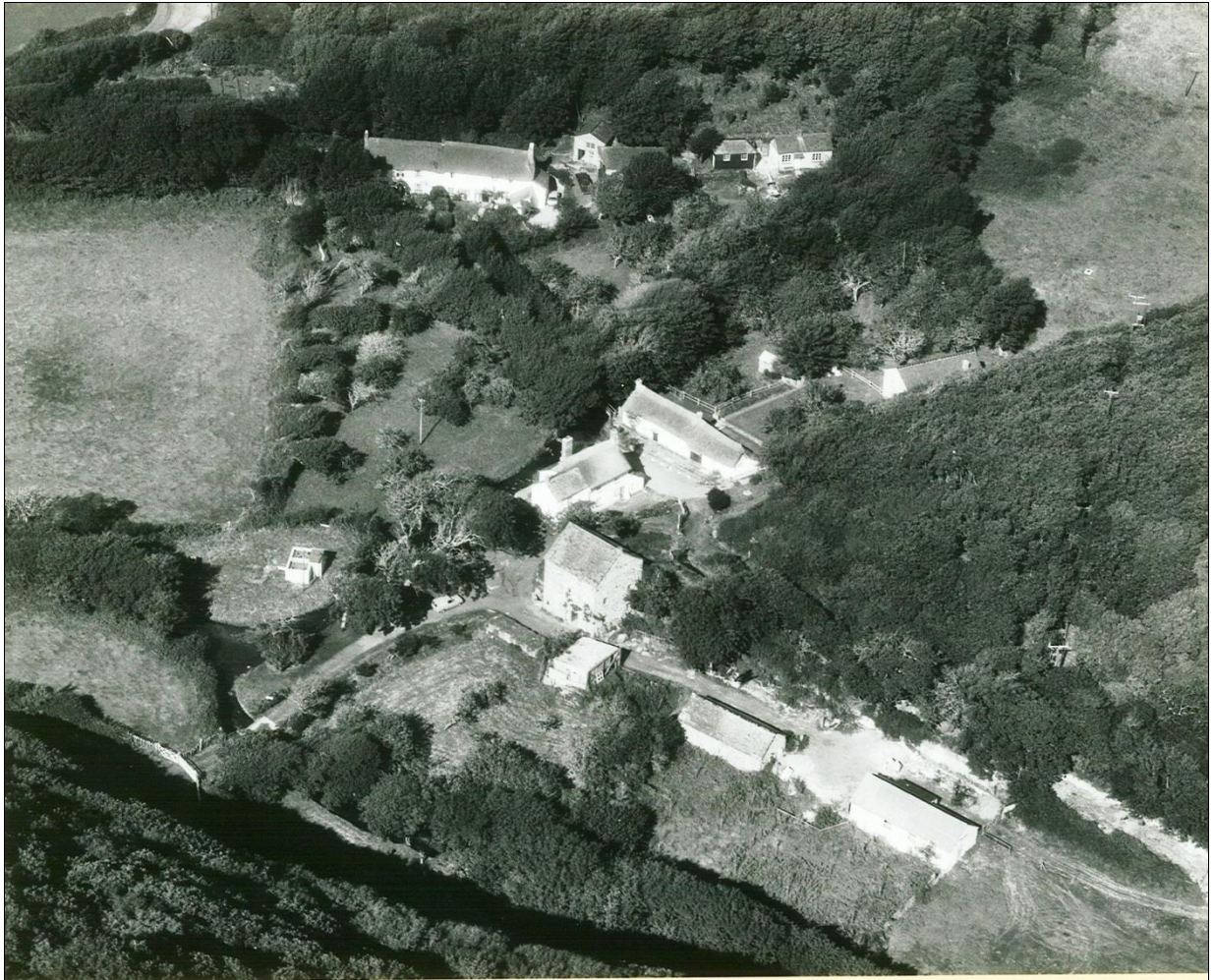
Coombe in 1969 when Landmark's repairs were in progress. The Mill House, Ford Cottage and the Carpenter's Shop are complete, work is underway on Chapel Cottage.
