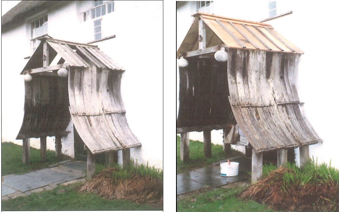
Canopy at no 1 Hawker's before and after 2004
