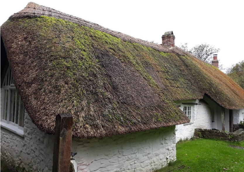
The thatch before (top) and after repair. As the front slope was in still good repair there was no need to renew it, apart from the protective ridge.
