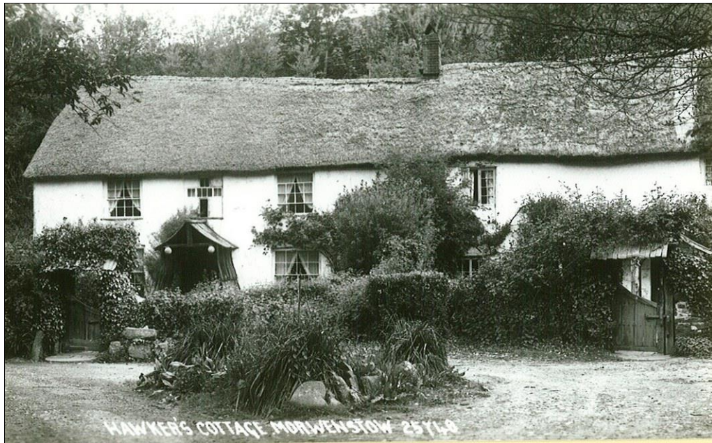
Hawker's cottage before restoration
