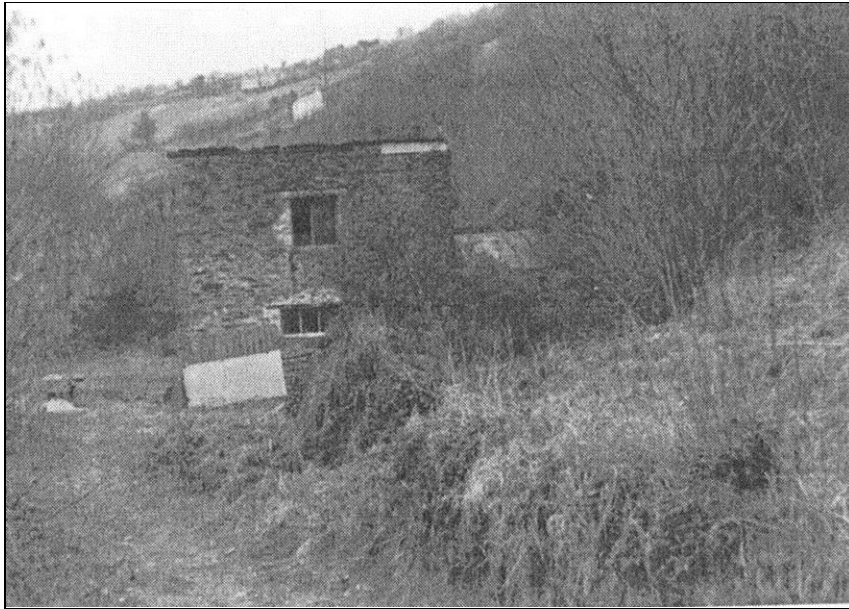
Crusher house looking up the valley.
