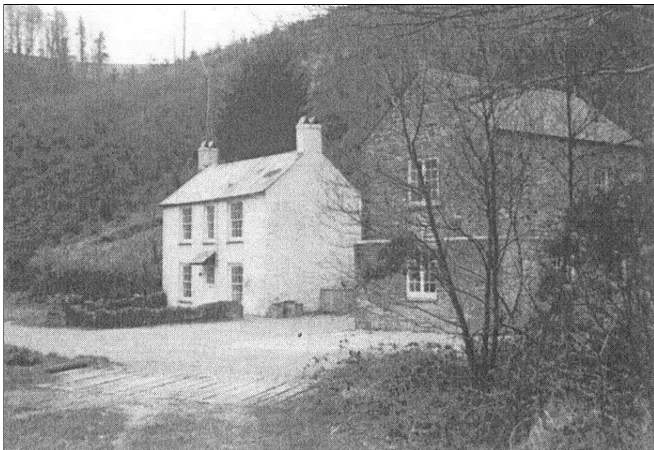
Mine Manager's Cottage and Engine House by Engine Shaft, restored by the National Trust.
