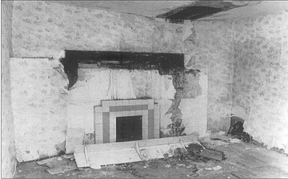
The sitting room fireplace before the partitions were removed during restoration
