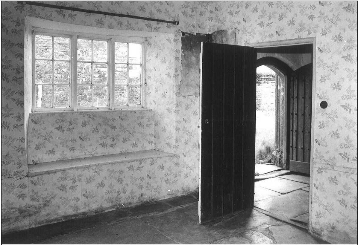
The sitting room before restoration
