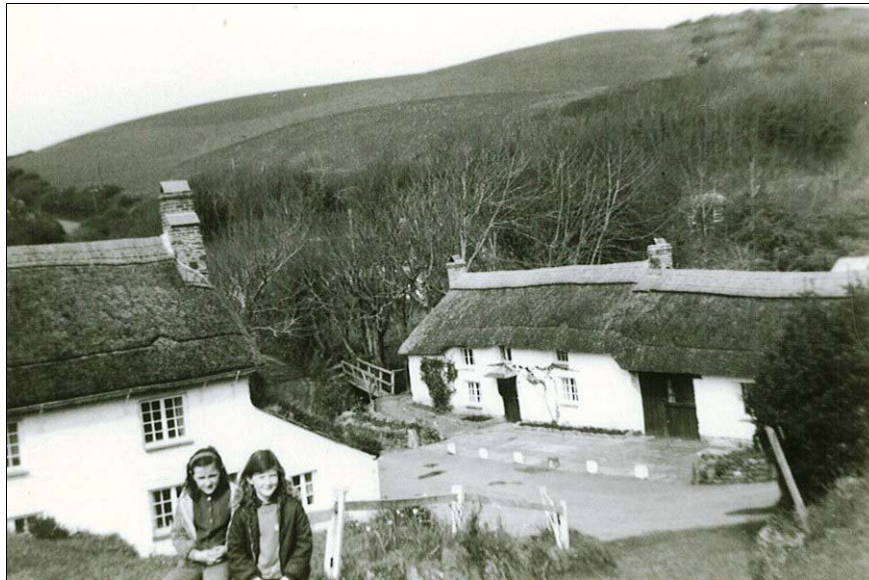
Ford Cottage after restoration
