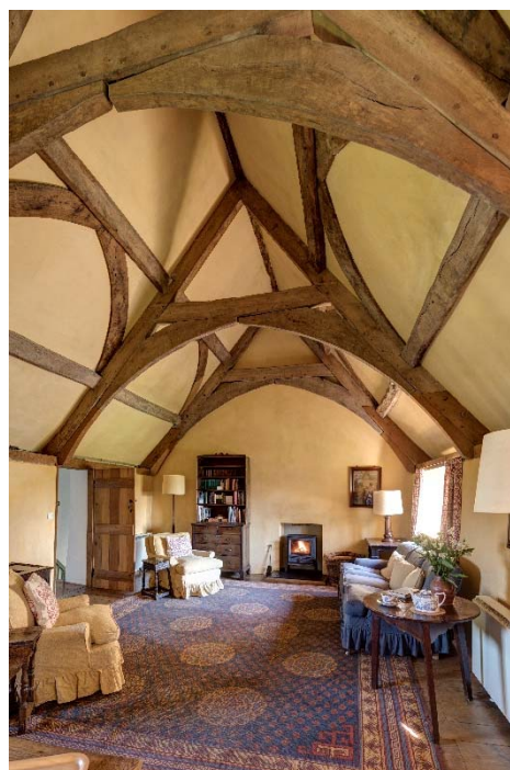
A view of the arch-brace trusses.
