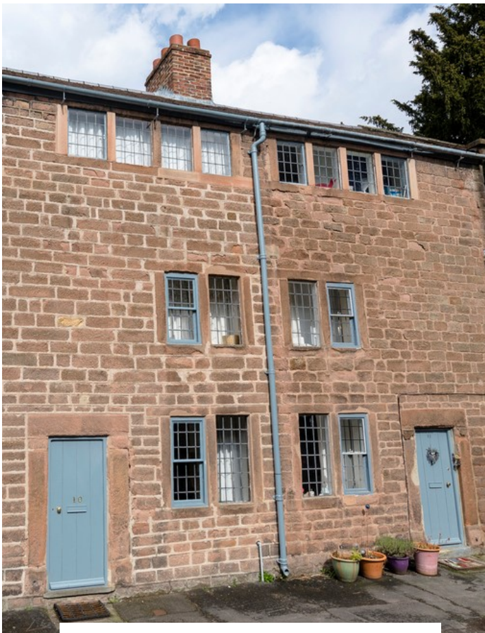
North Street as it appears today – note the long windows on the top floor to maximise light.
