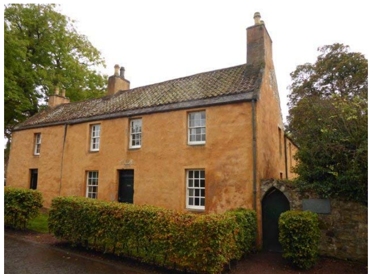
A picture of Collegehill House after it was restored in 2002.
