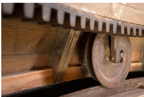
The giant cog mechanism which rotates to open up the observatory towers' roof.
