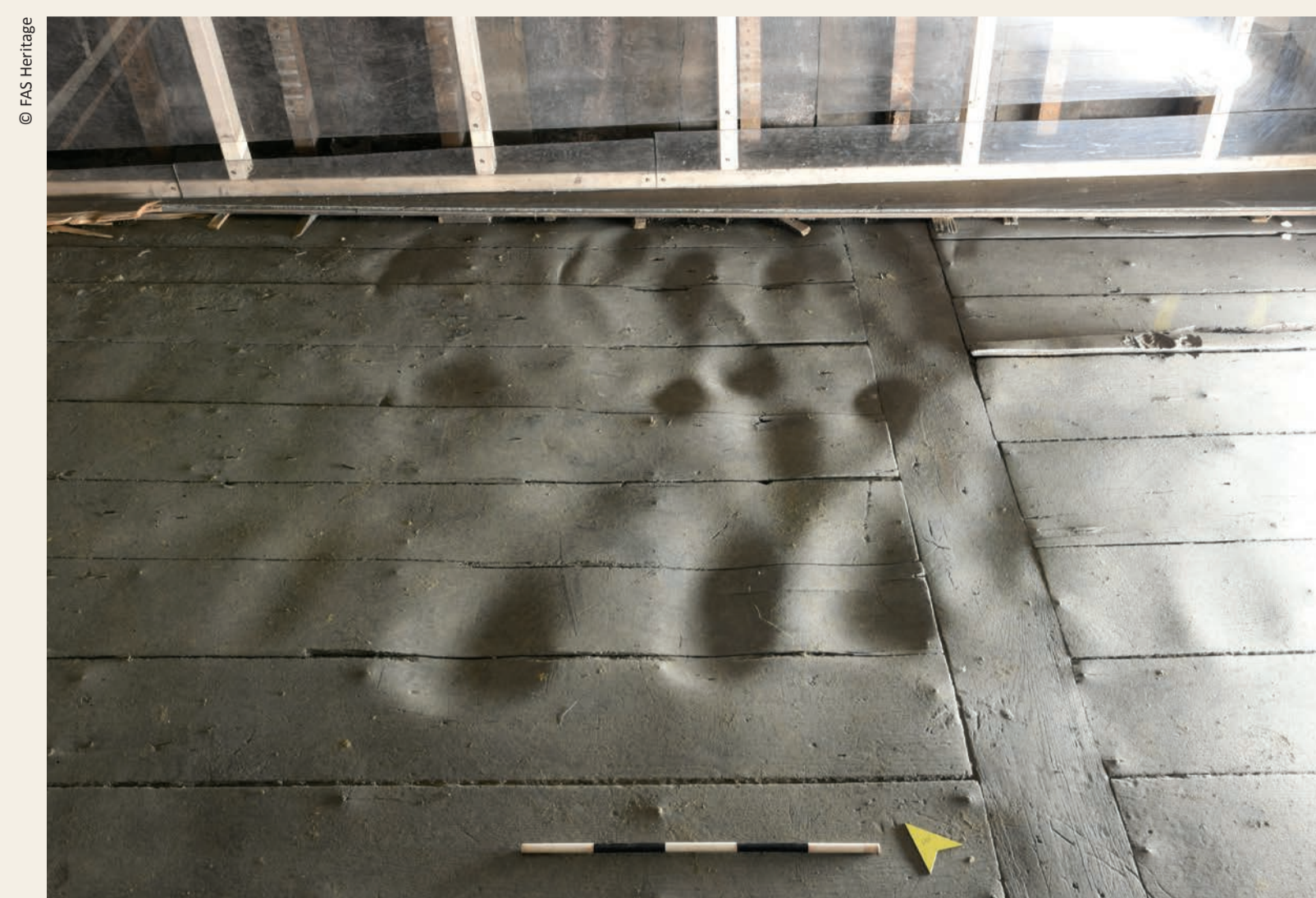
The floor of the Painted Chamber, showing signs of wear from the treadle of a loom or spinning wheel.
