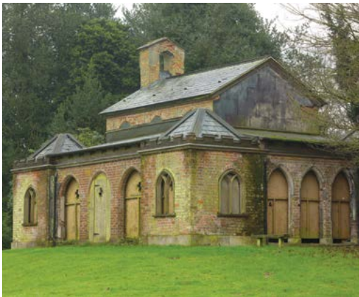
Cobham Dairy, Kent, built by James Wyatt in 1794, requires urgent support for the early phase of its restoration
