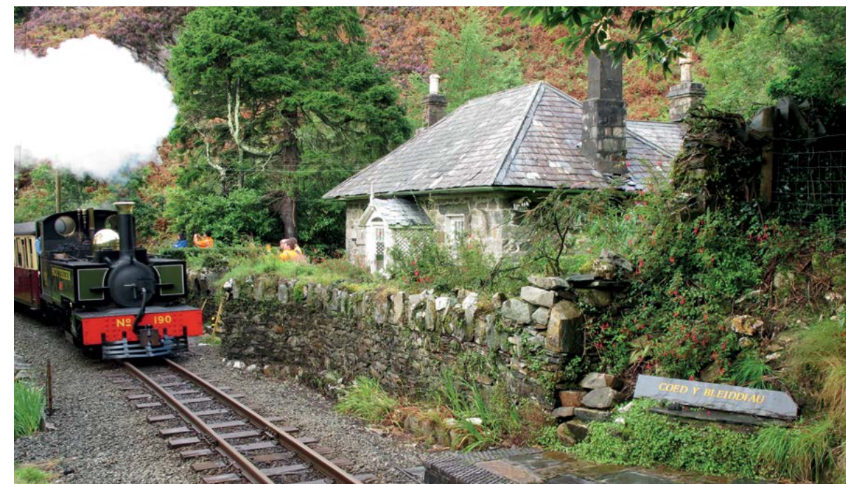
Coed y Bleiddiau before restoration. Guests will hear the nostalgic puff and toot of passing trains.
