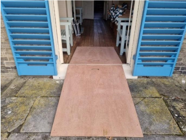
Image 15: A wooden ramp can be added to the Flower Room exit for step free access
